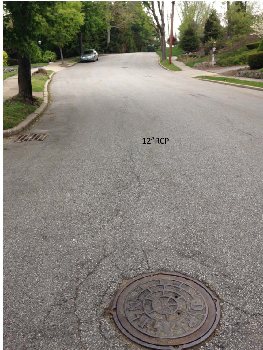
Downstream Drain Manhole & Proposed Pipe Alignment
